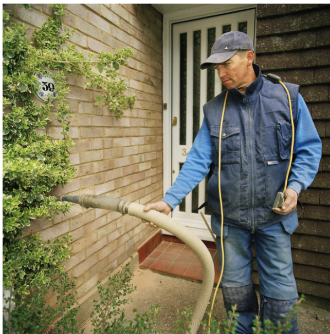
Cavity Wall Insulation is a straightforward, inexpensive job
